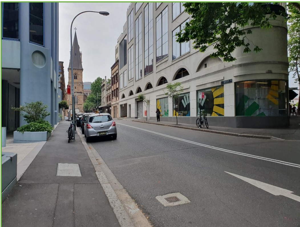
View looking east from intersection of Quay Street and Valentine Street
